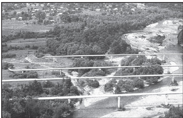
Fig. 8.17: Pipelines transporting natural gas in Ukraine
