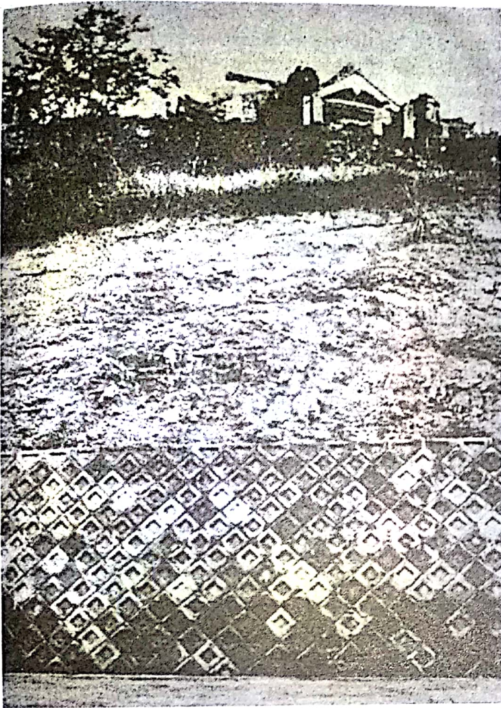
4.D An effective way of preventing landslide by building a concrete wall—Taiwan Goh Cheng Leong
