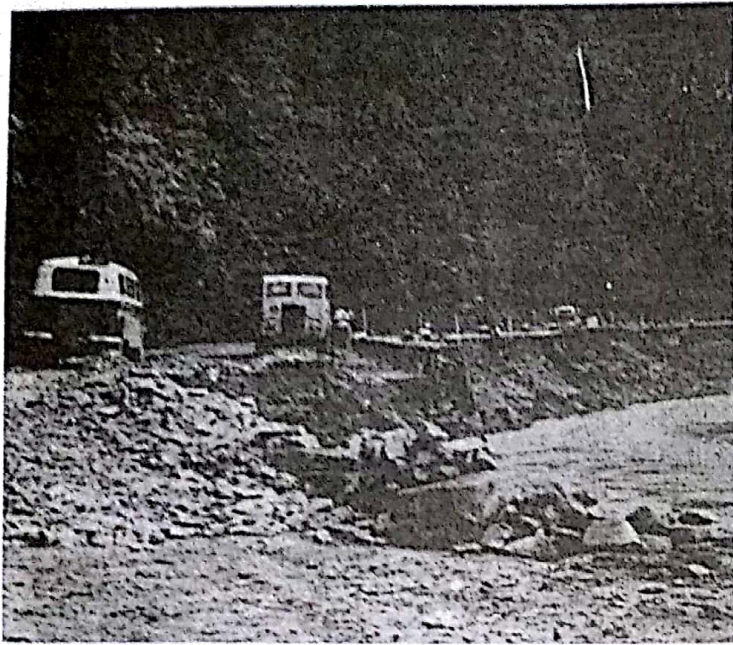
4.C A landslide after flood has damaged the road Jabatan Penerangan Malaysia
